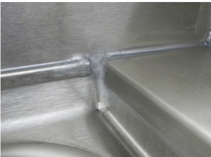
Soldered and Siliconed Seams
